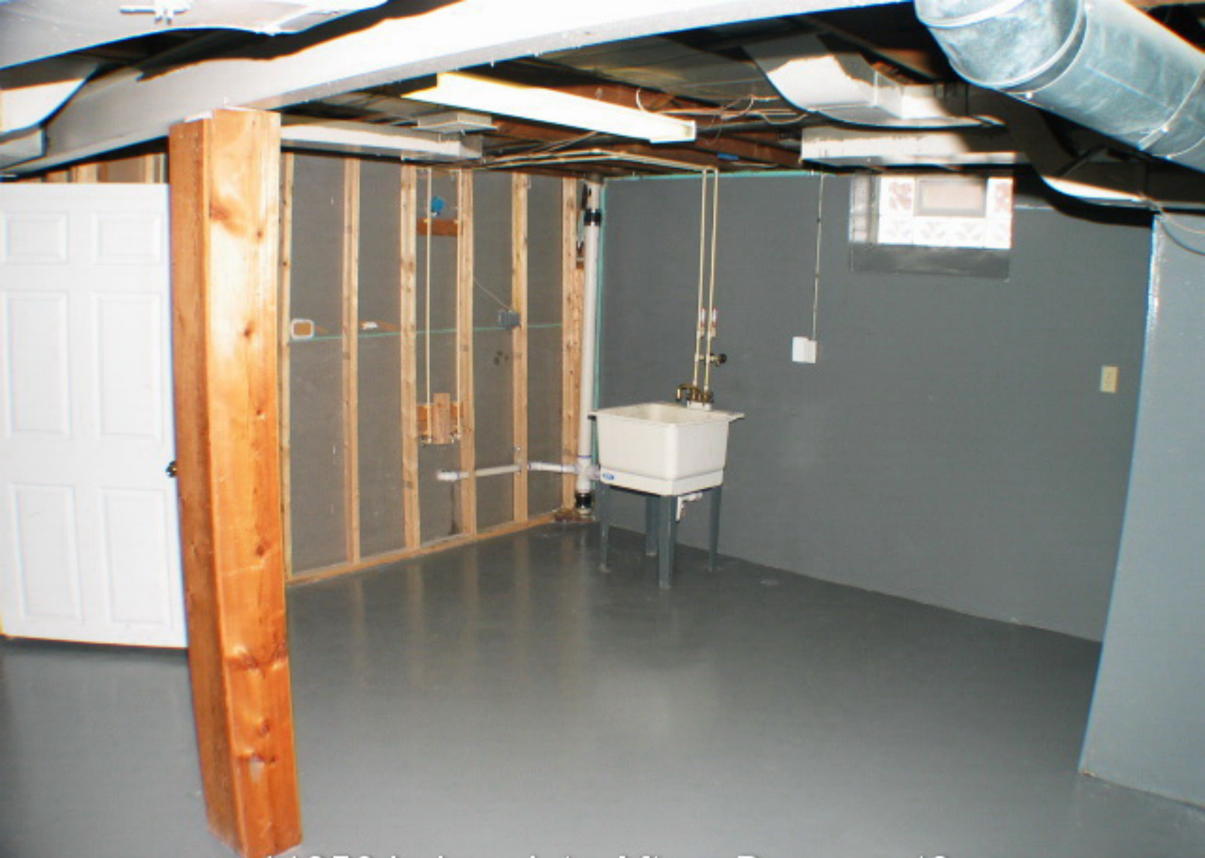
11058 Lakepointe After: Basement6
