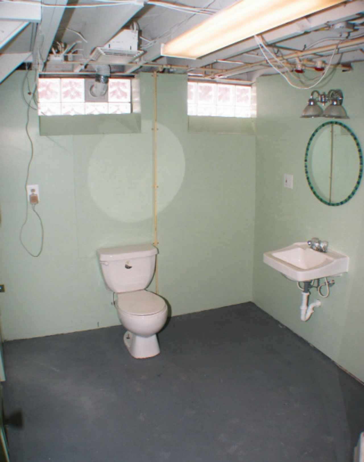
11058 Lakepointe After: Basement bath
