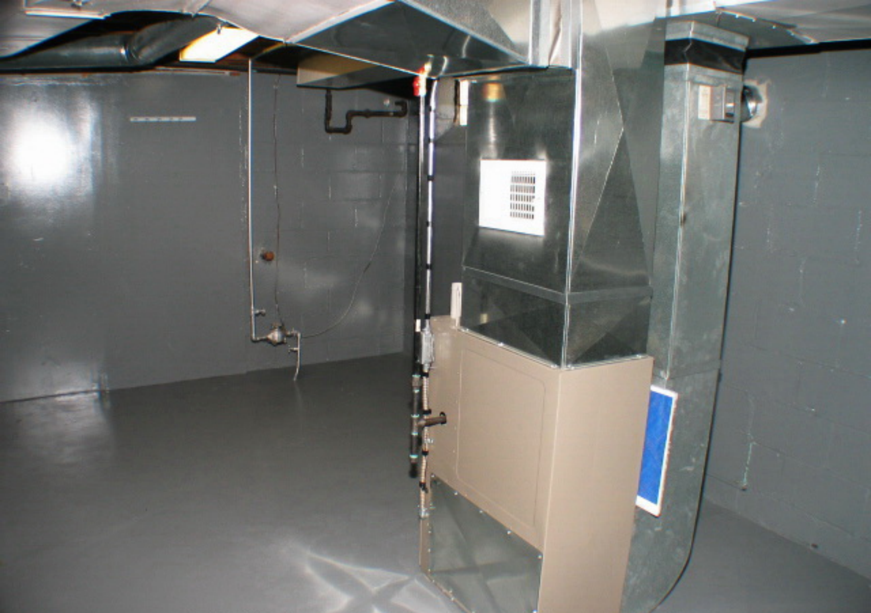
11058 Lakepointe After: Basement3
