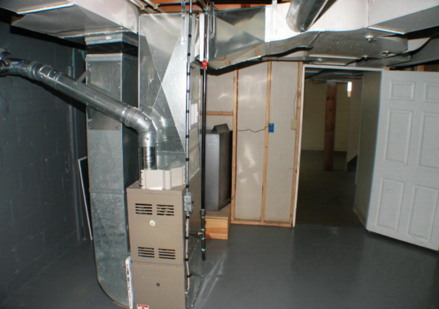
11058 Lakepointe After: Basement7
