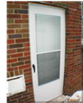
New exterior doors
