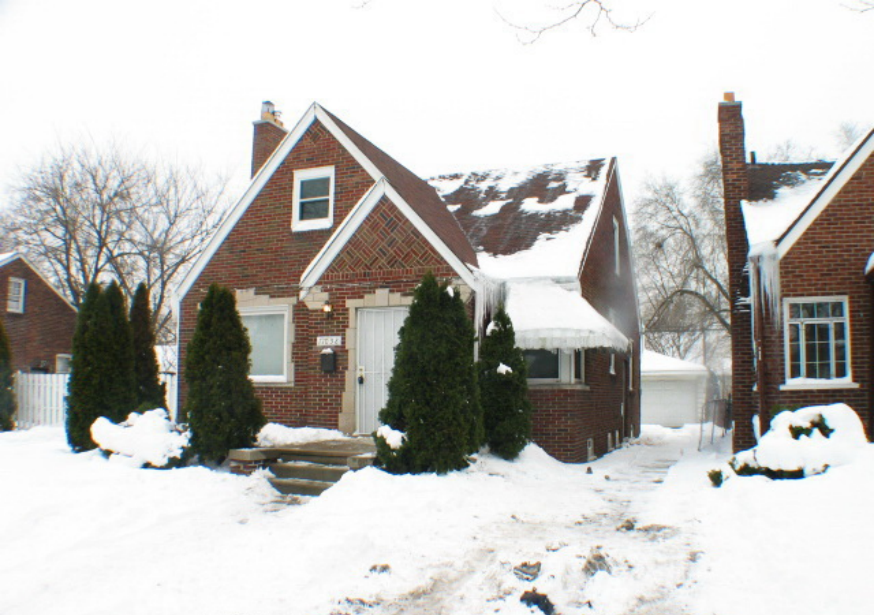
11058 Lakepointe After: South side
